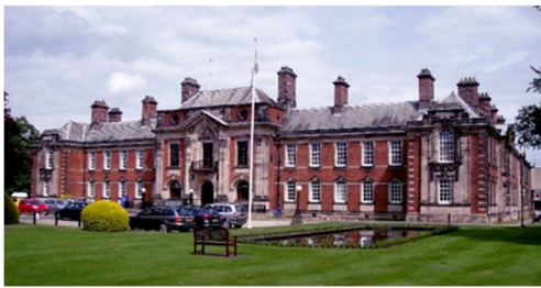
NYCC County Hall Brierley building
