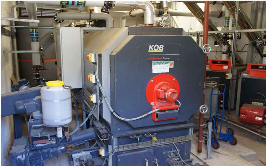
Installation of new biomass boiler Installation.
