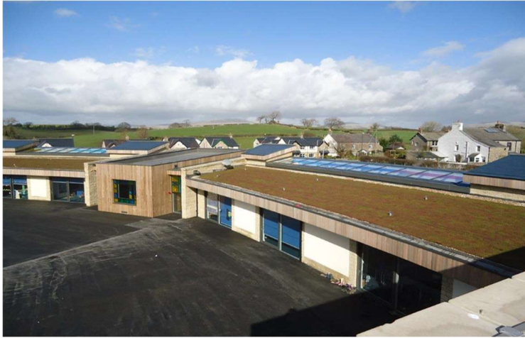
Bentham School – Indicating Sedum Roof.
