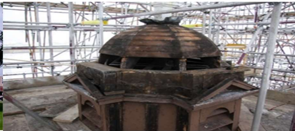
Repairs to the main roof dome
